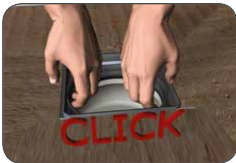
Step 7 Put your fingers through the drain hole in the shower tray ( ). Push down on the shower tray ( ) and pull the shower drain base ( ) upwards until it clicks into place into the drain hole in the shower tray ( ).
